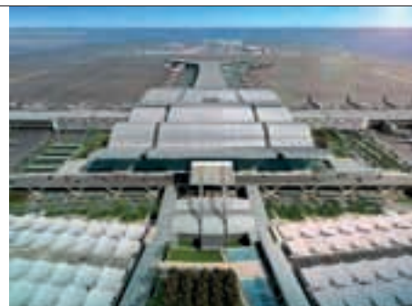
Photos: Doha airport
